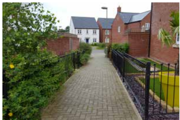
Pedestrian/ cycle cut-through, South West Bicester
