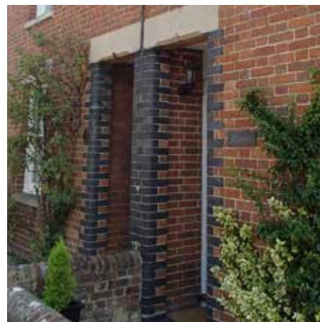
Localised brick detail around doorways
