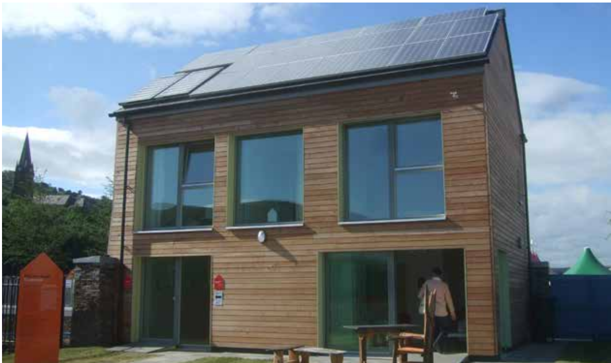
Larch House, Ebbw Vale is the UK's first zero carbon (code 6), low cost, Certified Passivhaus.
