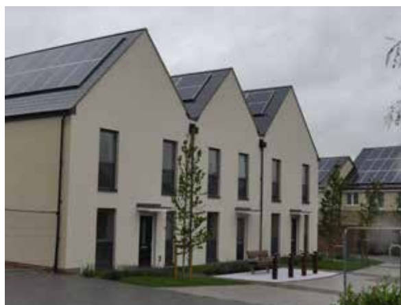
Bicester - Priory Road (top), Church Street (middle), Elmbrook, North West Bicester (bottom)
