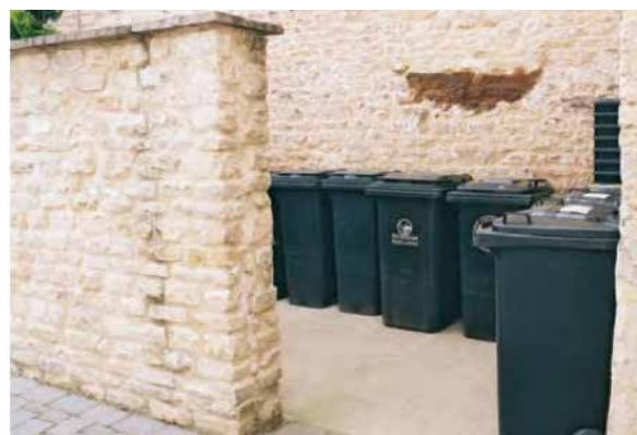
Example of an attractively designed bin store (source: West Oxfordshire Design Guide)
