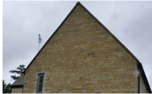
Steeply pitched roof with no overhang, Bletchington
