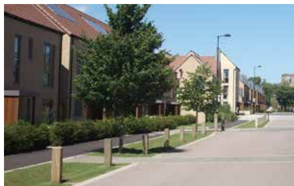
Incorporating SuDS along kerbside, Trumpington Meadows, Cambridge
