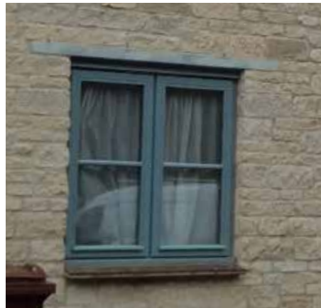
Casement window flush with wall, Bletchingdon
